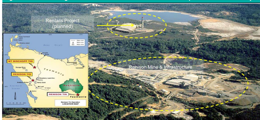
Figure 3 - View showing current Renison mine and infrastructure and planned Rentails facility
